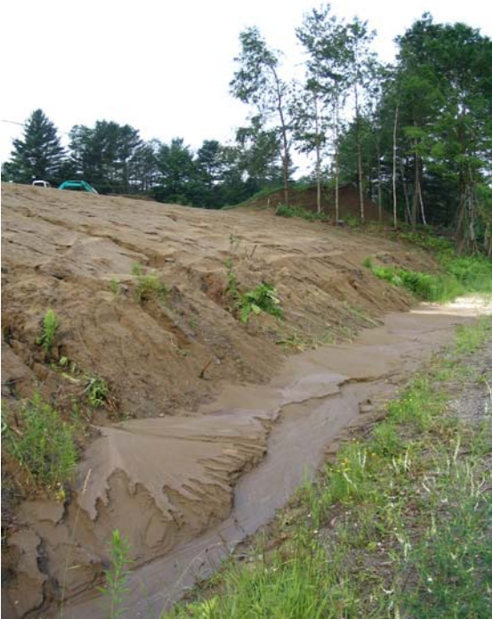
Construction site erosion and sedimentation
