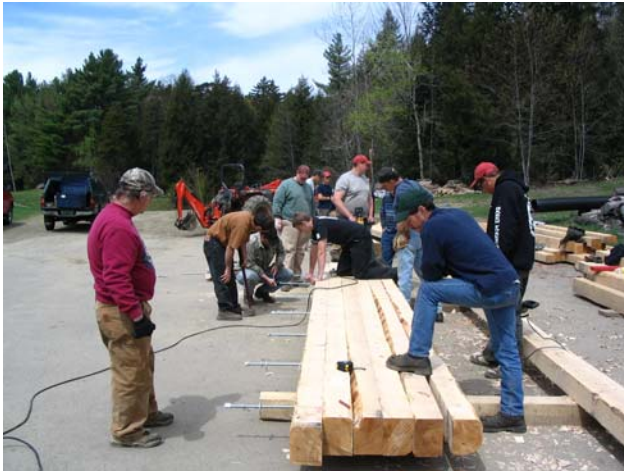
Portable Skidder Bridge construction workshop, Hardwick
